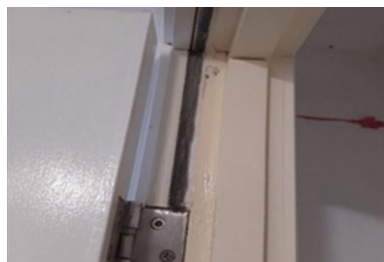
Combined intumescent strip/seal (frame fitting)
